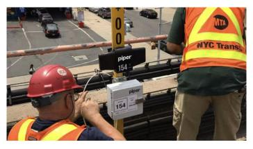
Piper team members were present in NYC and near the trackside during the wayside installation to answer questions and resolve issues quickly. Anchors were installed wayside of elevated tracks by being attached to survey markers. Anchors were also attached to predetermined locations in tunnels by Piper's custom developed bracketry.
