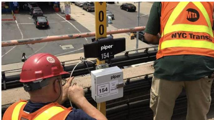
Piper team members were present in NYC and near the trackside during the installation process to address any questions and resolve issues promptly. Anchors were installed on the wayside of elevated tracks by attaching them to survey markers. In addition, anchors were attached to predetermined locations in tunnels using Piper's custom-developed bracketry.
